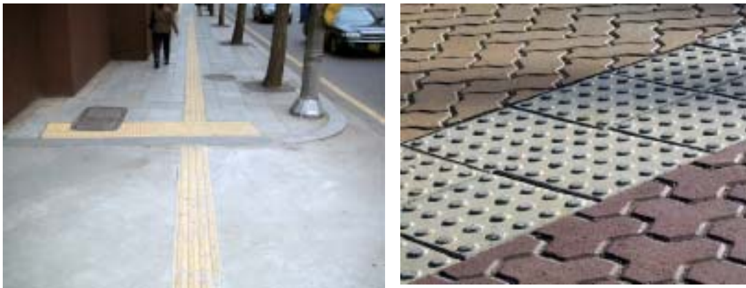
Photo 2 Tactile tiles (Seoul, The Republic of Korea)
